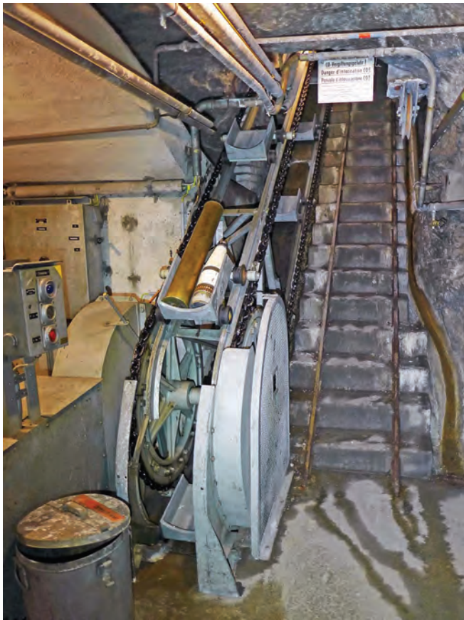
Fort San Carlo: The base of the slope shaft and ‘paternoster’ ammunition hoist to Turret 1. Note the lack of separation of shell and cartridge. Note also the carbon monoxide warning sign: gun crews were supplied with piped air
